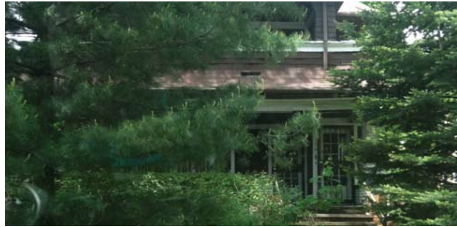
1724 Coventry Road deemed a public nuisance.
