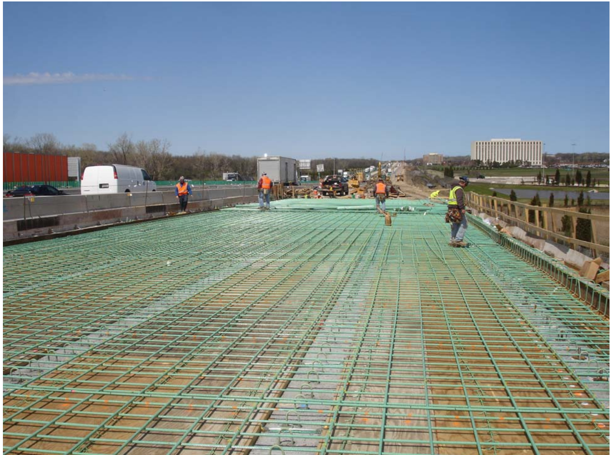
Figure 1 – Epoxy-coated reinforcing steel bar used in the deck of a bridge structure located in Illinois. (Photo Courtesy of the Epoxy Interest Group of CRSI)
