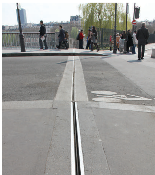
WR 50 joint Île Saint Louis bridge - Paris
