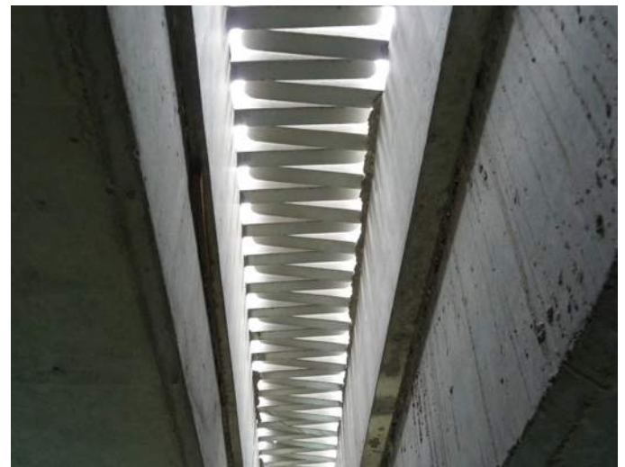
WP joint seen from below
