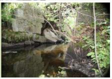
A survey of Pantry Brook and the adjacent area is needed to collect data to design the replacement Pantry Brook bridge abutments and for the design of the new bridge. A similar survey will be done at Hop Brook, but those abutments are intact and will not need replacement. The flood plain elevations adjacent to both brook crossings will be delineated. This survey work is actively in progress.
