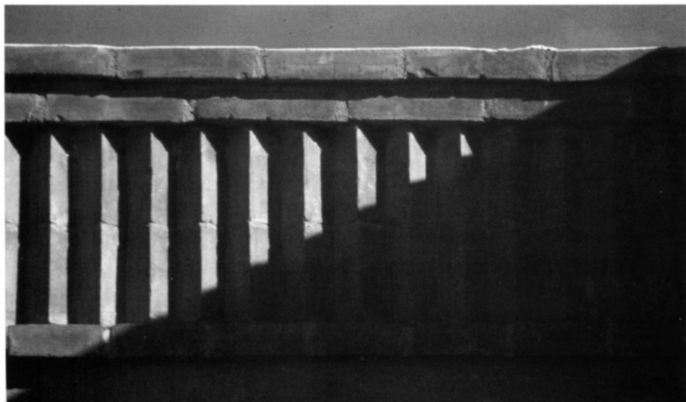
Frieze, Caldwell Residence, Tucson Arizona, 1940. The Mudéjar decorative brick tradition continued into the Spanish Colonial Revival period. (Photo by author)
