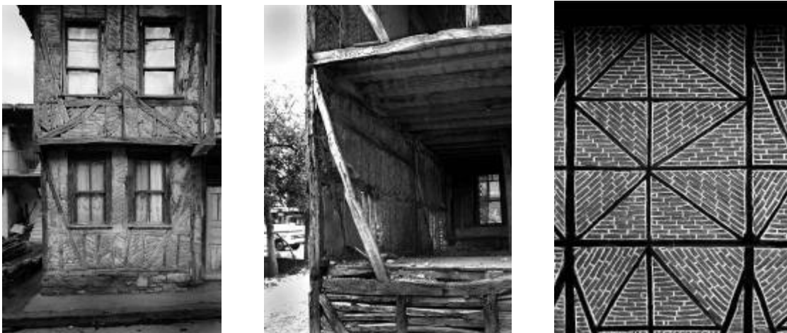
Figure 7: (a) Himis house in Gölcük damage district after the 1999 earthquake with no visible damage.
