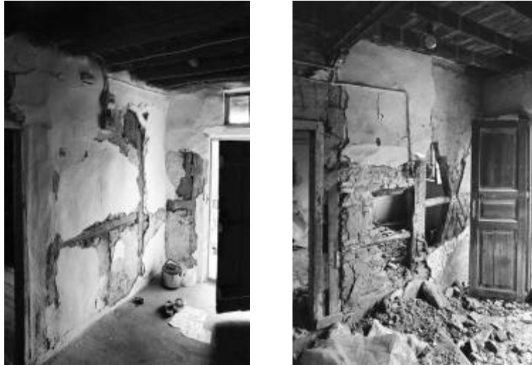
Figure 8: (a) Interior of himis house in Orta after 2000. (b) Interior of himis house in heart of damage district in Adapazari after 1999.
