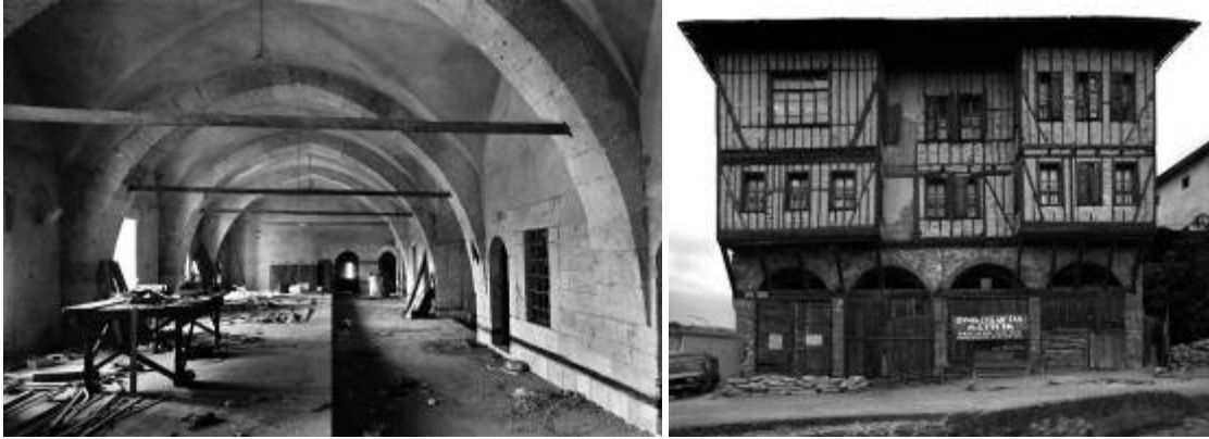
Figure 6: (a) Caravansary, Safranbolu, Turkey showing timber hatil in bearing wall masonry visible on right at base of wall, 2000.
