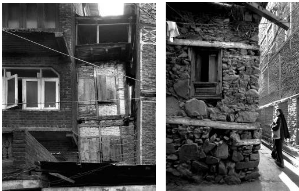
Figure 17: (a) Remnant of a traditional house in Srinagar, Kashmir in 2005. (b) An historic house of Taq construction still extant in Srinagar in 2005.
