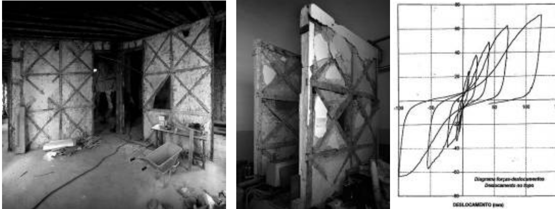
Figure 12: (a) 18th Century building in central Lisbon showing “Pombalino gaiola ” construction, 2003. (b) Gaiola wall sections from a late 18th or early 19th C. building after having been tested. (c) Hysteresis diagram from one of the wall tests of the walls in figure 12b.
