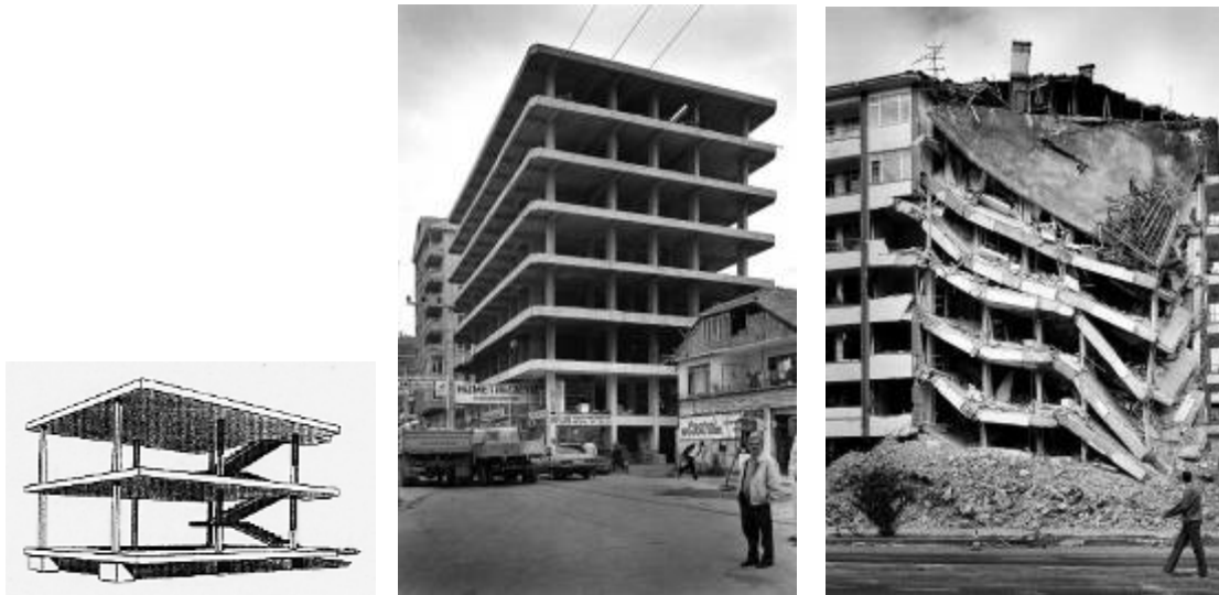
Figure 15: (a) Le Corbusier's conceptual Dom-Ino House, 1915 (b) Building under construction in Gölcük at time of 1999 earthquake (c) Partially collapsed reinforced concrete infill-frame building in Gölcük, 1999.
