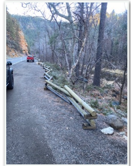
This is logworm fencing
