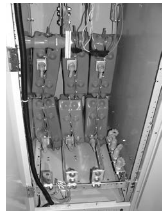
Grounding Balls and Covers
