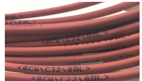
Control Wire Marking
