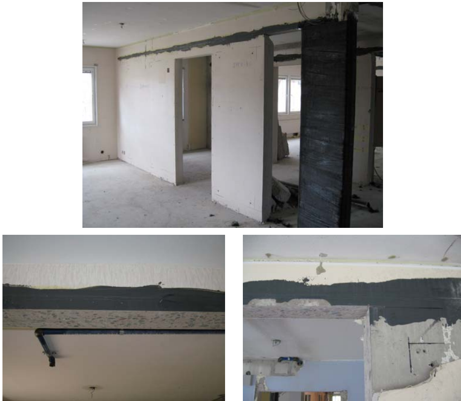
Figure 5-10: Photographs from the application of the strengthening system
