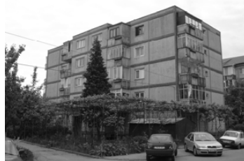
Figure 1: Typical PRCLP building
