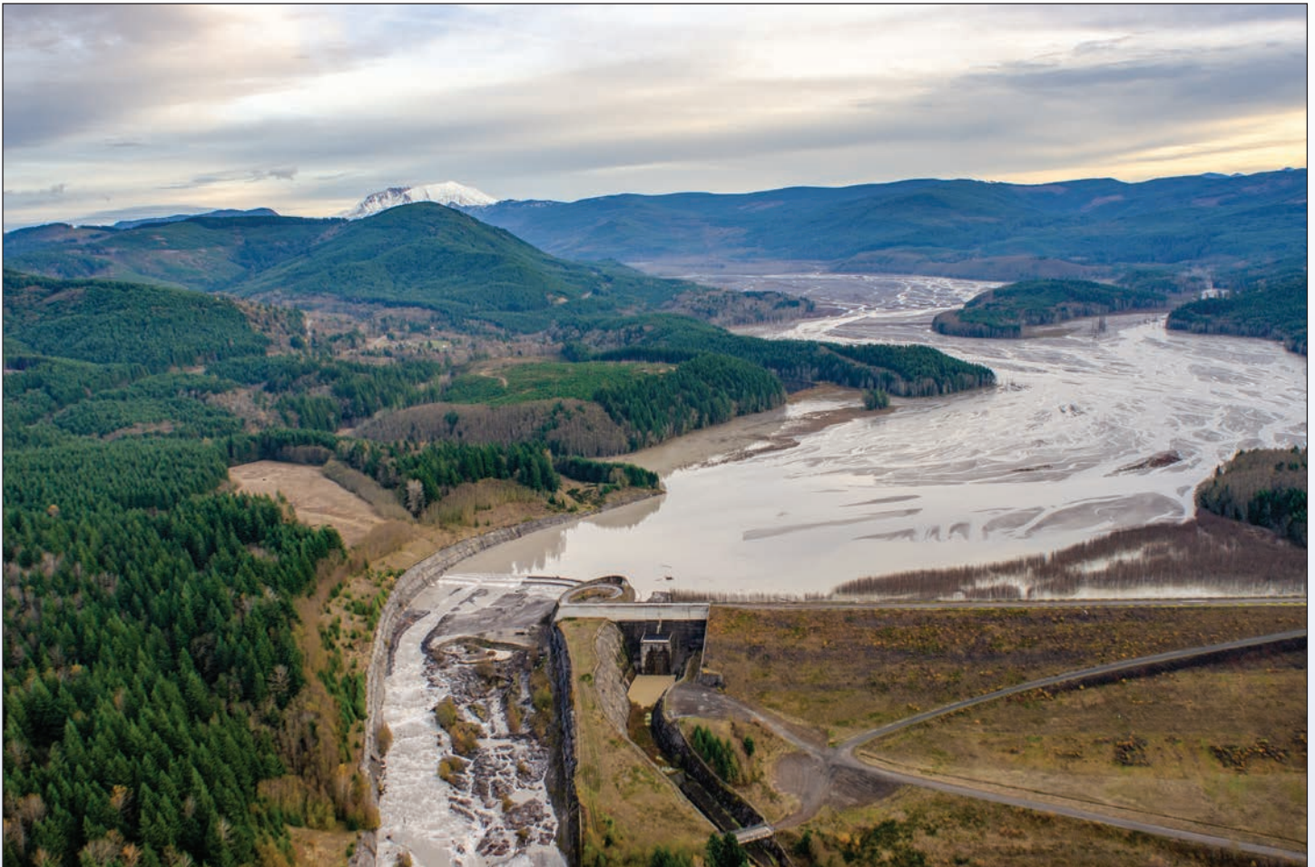
Photograph of the sediment retention structure (SRS) on the North Fork Toutle River after the 2012 spillway was raised. View is upstream to the east. Photograph by Adam Mosbrucker, U.S. Geological Survey.
