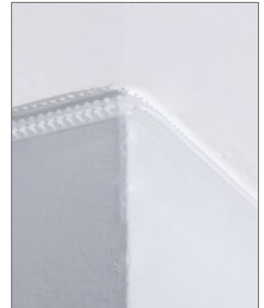
Clear Track Hallway Fibre Pathway Installed Around Exterior Corner
