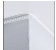
Clear Track Hallway Fibre Pathway
