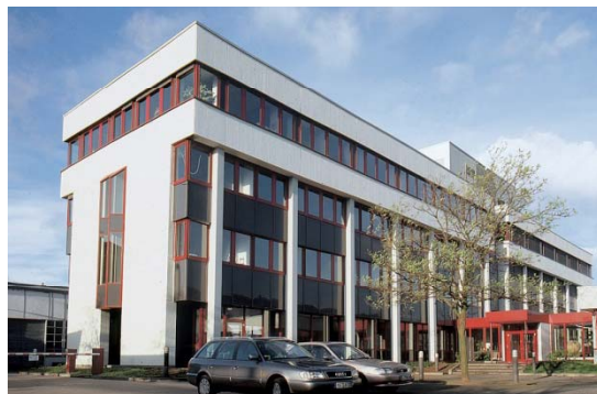
Modernisation of holding building
