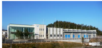
Hydrogen Energy Test & Research Center (HyTReC)
