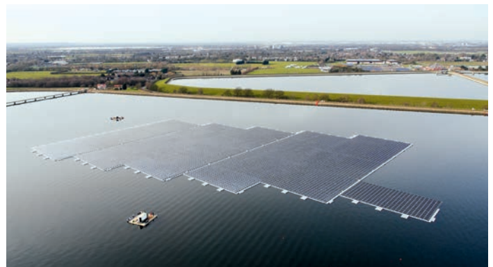
Above: Lightsource BP’s floating solar farm near London in the UK.
