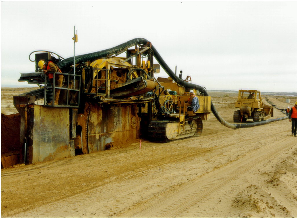
Figure 5.—Installation of drain pipe (without geotextile sock) using wheel trencher equipment.
