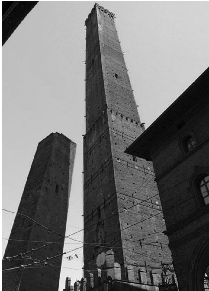
FIG. 1.3 Tilting of Garisenda Tower (left) and Asinelli Tower (right) in Bologna, Italy (Courtesy of Braja M. Das, Henderson, Nevada)
