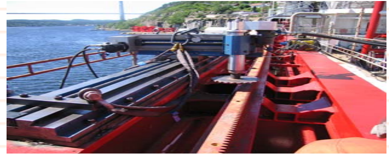
Milling of crane beam (30m)
