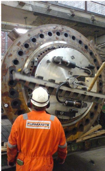
Machining on heat exchanger
