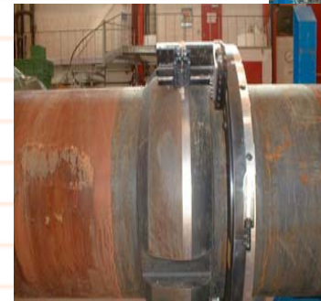
Axial turning with a pipe cutting machine
