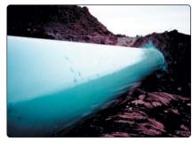
Pipe rehabilitation project completed using 3M 6 Scotchkote coating — and repaired with Scotchkote hotmelt patchsticks.
