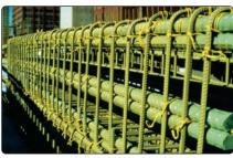
Rebar coated with 3M™ Scotchkote™ 413.
