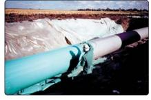
3M™ Scotchkote™ liquid epoxy being applied 21 to a pipe for a rehabilitation project.
