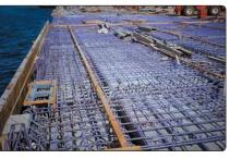
3M™ Scotchkote™ 426 coated rebar in naval pier prior to concrete pour.
