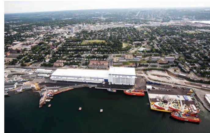
At 408 metres in length, the Assembly and Ultra Hall is the equivalent of nearly 7 National Hockey League (NHL) ice surfaces
