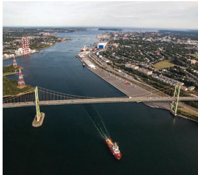
At 46 metres in height, the Assembly and Ultra Hall would just clear under the Halifax Harbour Bridges
