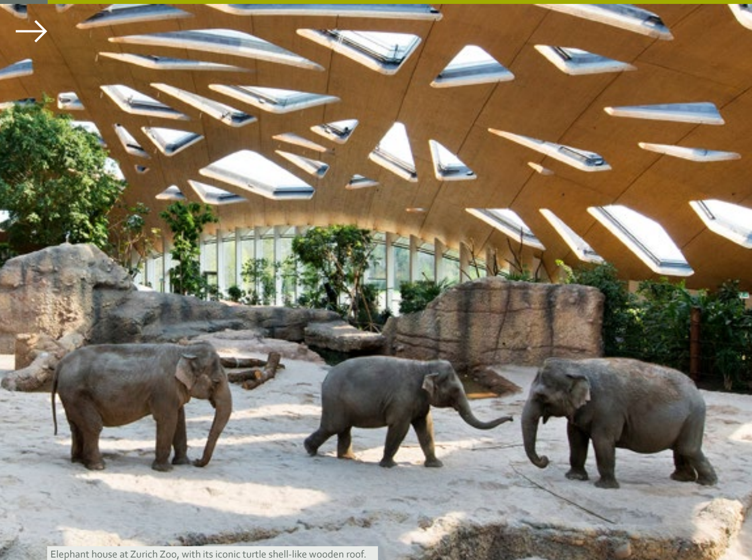
Elephant house at Zurich Zoo, with its iconic turtle shell-like wooden roof.
