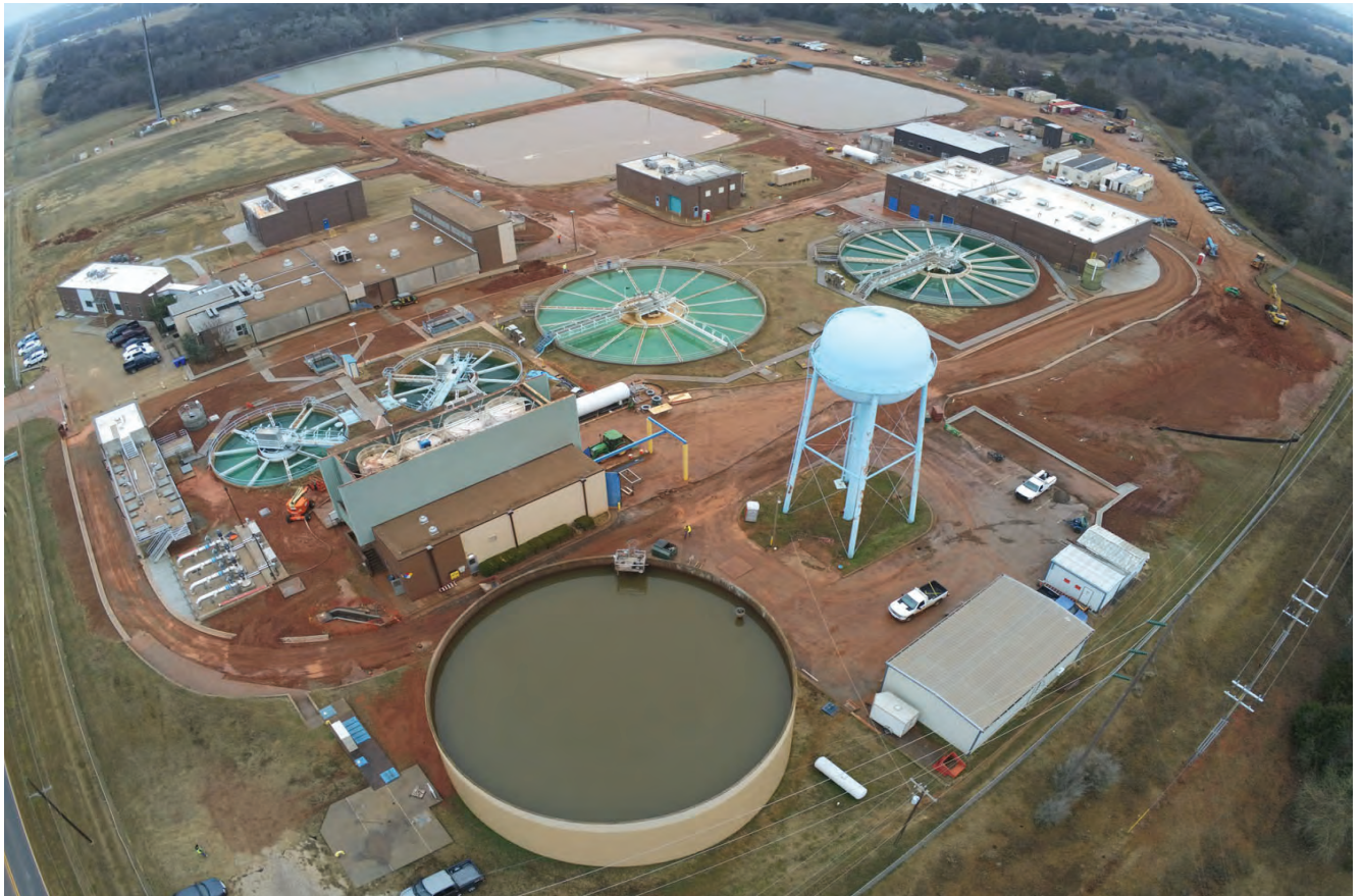
Improvements to Norman Water Treatment Plant
