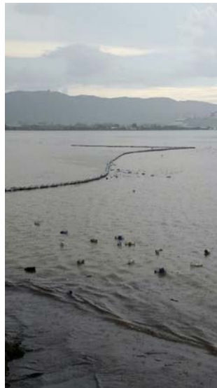
The anchor rope for the boom came lose due to storm surge during a heavy rainfall event on October 28 th , 2015. Since this picture was taken the boom has been repaired.
