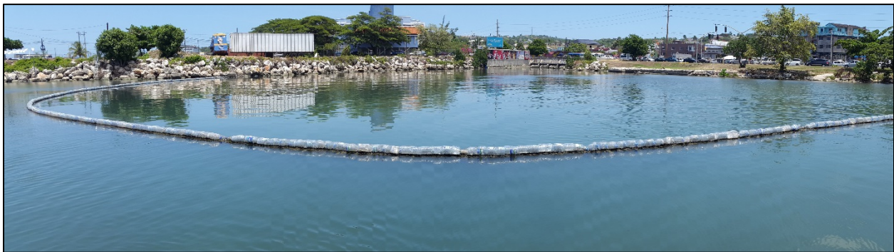
Figure 7: The South Gully Debris Containment Boom (DCB)
