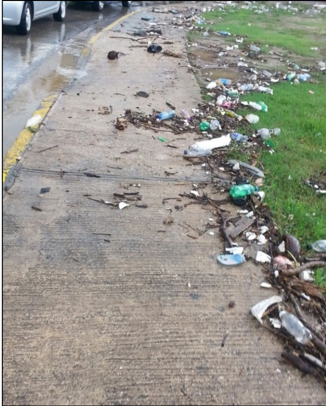
Figure 9: Garbage litters a section of Howard Cooke Boulevard in Downtown Montego Bay after heavy rainfall flooded drains
