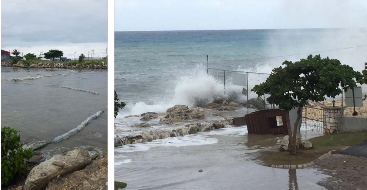
Left: Damage to the boom caused by the severe weather January 21 st – 22 nd , 2016. Right: storm surge on January 21 st , 2016 at the gate to Pier One.
