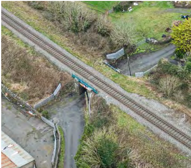
Stone bridge at L71051
