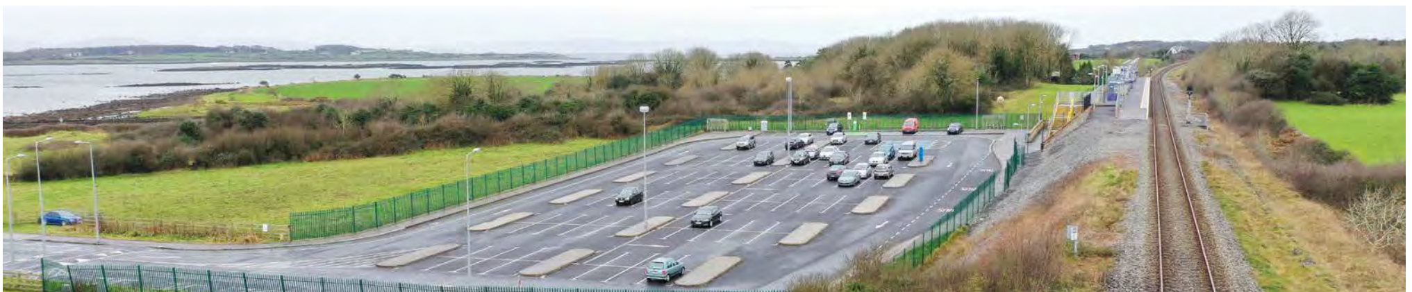
Existing carpark, railway station and single track railway
