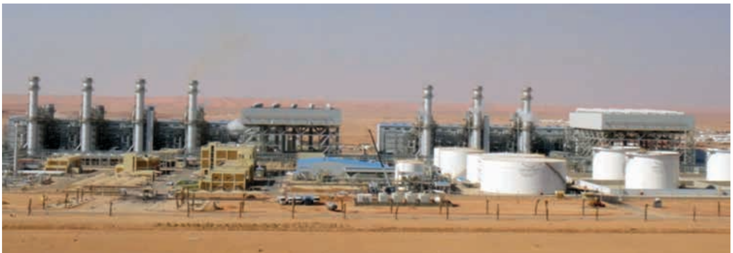
Figure 17 - PP11 combined cycle power plant
