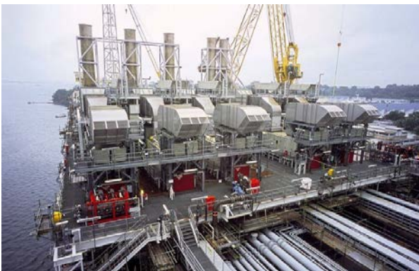
Figure 18. Gas Turbine Installation on an FPSO
