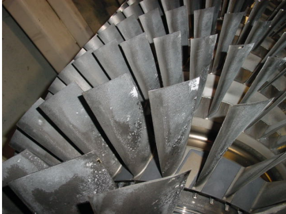
Figure 4. Salt Deposits on Compressor Blades (Courtesy, Turbotect Ltd.)
