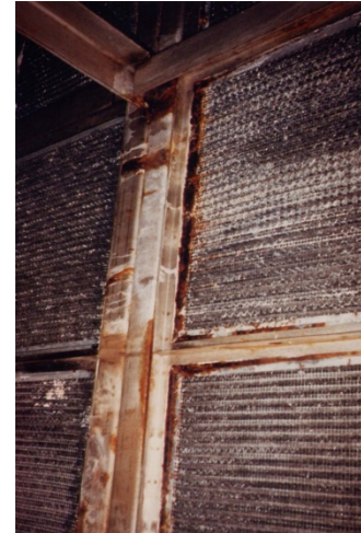
Figure 34. Salt Leeching Through Intake Filter (Clever, 1990).
