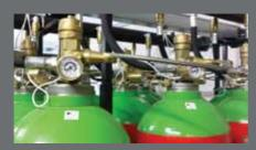
i-Flow systems eliminate the peak pressure point and achieve a balanced, constant flow during release.
