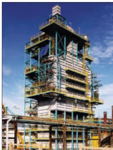
Ethylene Cracker Unit
