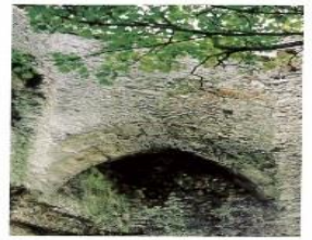
A surviving latrine outlet, which spans the angle of the inner bailey wall and a Roman bastion
