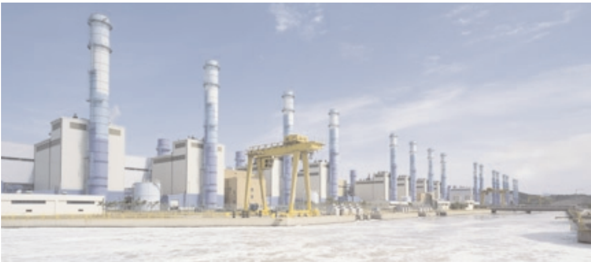
Figure 47. 4000 MW multi-shaft STAG installation
