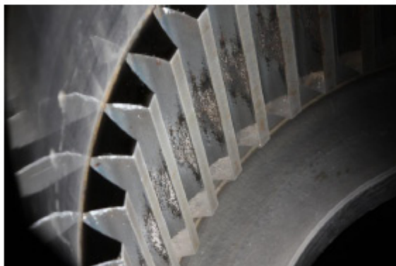
File Name: IMG_6244.JPG Comments: Hollow shaft spline fretting. Looking toward generator.
