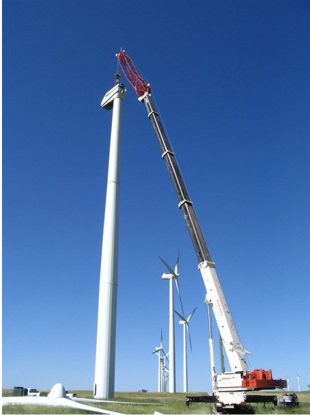
Figure 12. GRC gearbox installation in Ponnequin (NREL PIX/19257)
