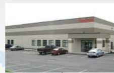
ThreeBond International, Inc. (Moraine Plant)
