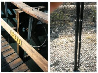
Figure 2.17 - Pond Electrode with Sub-Electrodes Placed Directly in Seawater with Wooden Fence to Avoid Transfer Potentials
