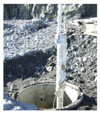
Figure 5.40 - Electrode element and encasement well
