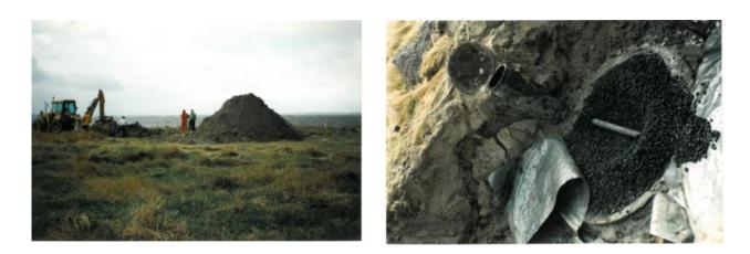
Figure 2.15 - Beach electrode in coke with covers to avoid Mixing of coke and soil
