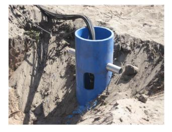
Figure 2.8 - Completed sub-electrode assembly before inserting Vent pipe and filling with coke
