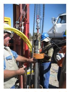
Figure 2.7 - Assembly of sub-electrode element FOR Vertical Well type Electrode
