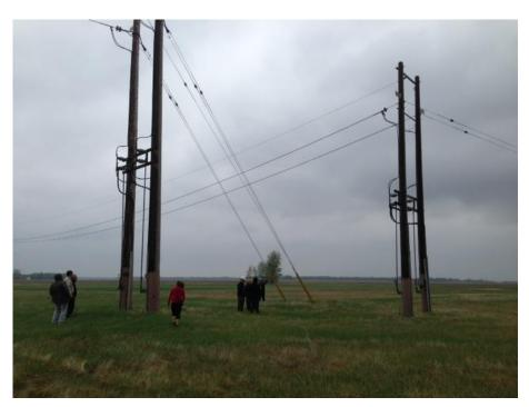
Figure 7.4 - Electrode Site without Fence and Electrode Switches Mounted on Distribution poles
