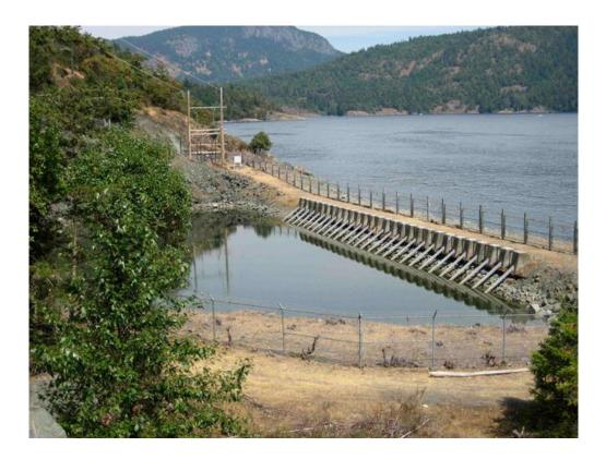
Figure 5.33 - Electrode Elements Arranged on Inside of Breakwater
