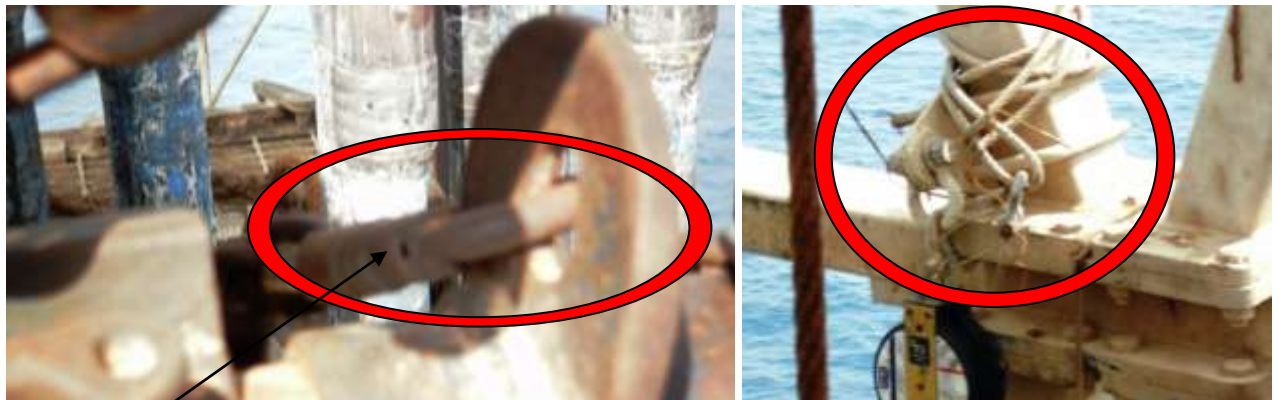
7- A carabiner was in use at the monkey board as part of lifting gear attachment. This should be removed and only the properly rated shackles should be in use as connectors. Seen above is also derrick-mans SALA with no color coding of block, sling or shackle.
