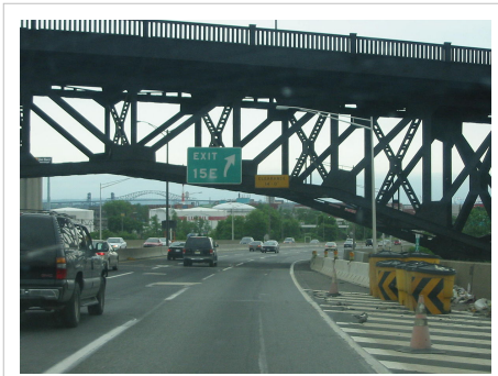
The New Jersey Turnpike, as seen in 2004 before it was lowered as part of a seismic retrofit and widening project, passes under the skyway.
