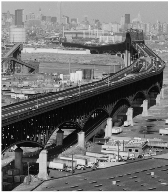
View looking east in 1978 photo from Historic American Engineering Record Survey, NJ-34 showing the South Kearny center ramp. Built to promote industrial development, it proved to be too dangerous for trucks.
