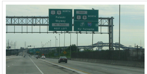
US 1/9 is elevated on embankments through eastern Newark; the skyway (background) rises higher to clear the Passaic River.
