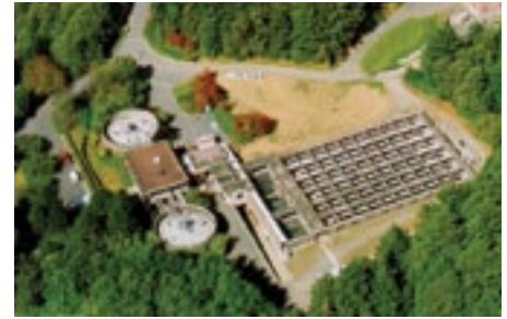
Figure 7. The Greater Nanaimo Pollution Control Centre uses biogas from wastewater treatment, and operates a cogeneration unit with a capacity of around 300 kW. Source: Regional District of Nanaimo.
