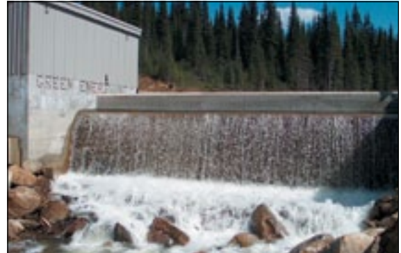
Figure 10. Hystad Creek small hydro project near Valemount.
