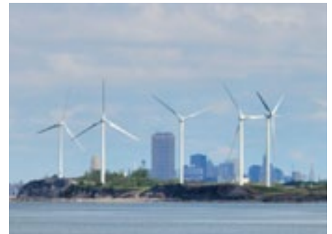
Figure 18. Coastal turbines mounted on flat ground, more than 10 m above any nearby physical barriers, with substantial setbacks from other buildings.
