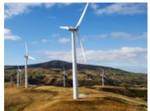
Figure 19. Example of a ridge-mounted wind turbine. Note gently rolling ground and lack of obstructions.
