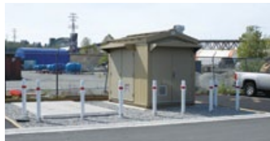
Figure 13. A 23 kW PRV Hydro project, recently constructed in the District of North Vancouver.
