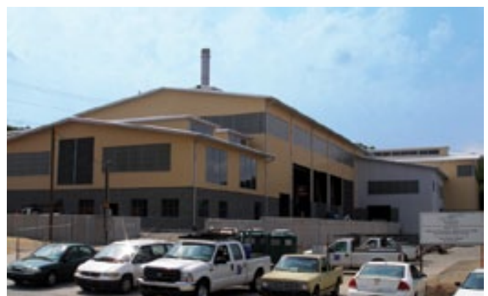
Figure 23. University of South Carolina's gasification system. Source: Nexterra Systems Corp.
