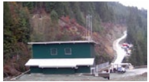
Figure 11. A Powerhouse for a 5-10 MW hydro project. Courtesy of Cloudworks Energy Inc.
