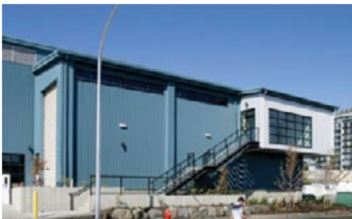
Figure 22. Dockside Green's gasification system is housed in a building designed to fit right into the urban neighbourhood. It provides heat and hot water via a district heating system. Source: Nexterra Systems Corp.
