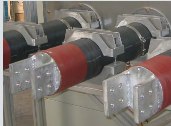
Fig. 18 Fully-insulated busbars – horizontal connection
