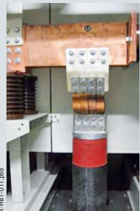
Fig. 20 Fully-insulated busbars – bottom connection
