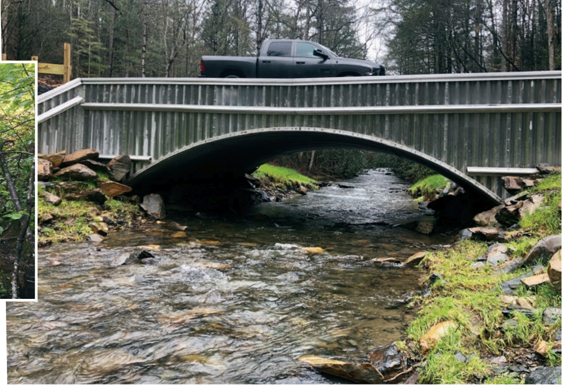
THIS PAGE Before and after. Collapsing and perched culverts at Mill Creek in the Chattahoochee National Forest limited fish passage for important species. TNC and partners replaced them with a bottomless culvert. © Katie Owens/TNC LEFT PAGE A student works with professor Troy Keller (in the stream) to monitor aquatic species after the removal of two dams near Fort Benning. © Henry Jacobs, HJacobs Creative
