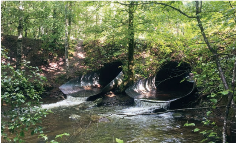
THIS PAGE Before and after. Collapsing and perched culverts at Mill Creek in the Chattahoochee National Forest limited fish passage for important species. TNC and partners replaced them with a bottomless culvert. © Katie Owens/TNC LEFT PAGE A student works with professor Troy Keller (in the stream) to monitor aquatic species after the removal of two dams near Fort Benning. © Henry Jacobs, HJacobs Creative
