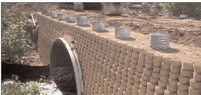
Stacked Cellular Confinement Facing
