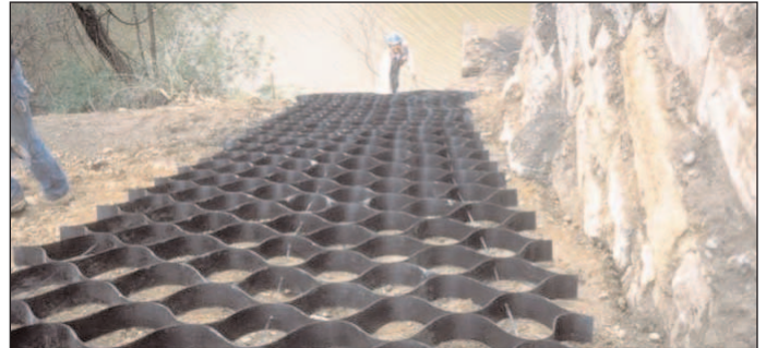
Cellular Confinement Stabilization
