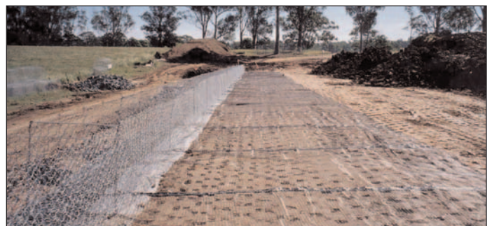
Gabion Basket Facing
