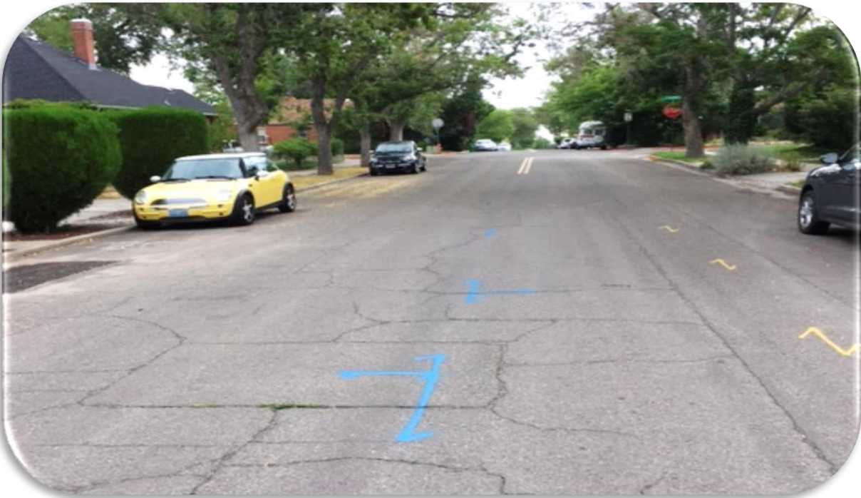
Photo #2 – Walker Avenue. Note Block Cracking
