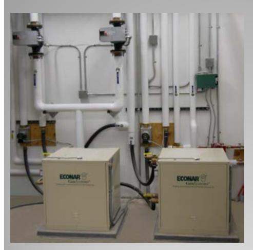
2 X 8T Hydronic "Heat Only" GSHP System Served by Integrated 2 X 8T Horizontal Slinky GHEX.
