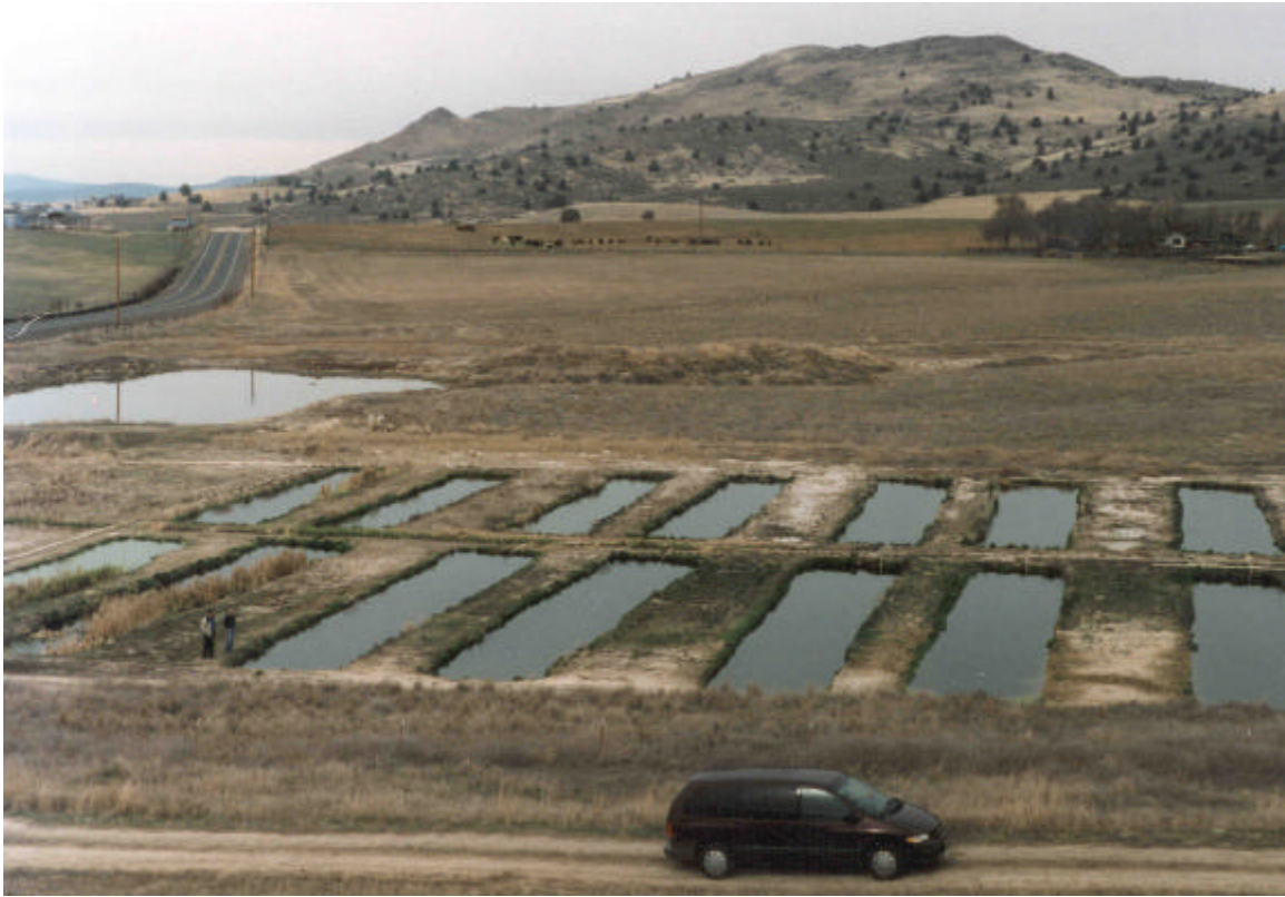
Overview of the 72 15-ft x 100-ft fish ponds near Klamath Falls, OR.
