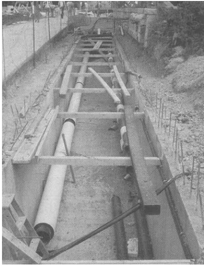
Figure 4. View of the tunnel under construction.
