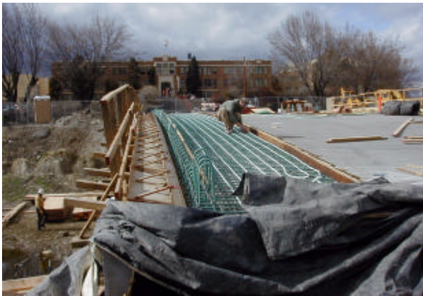
Figure 5. Bridge sidewalk loops.
