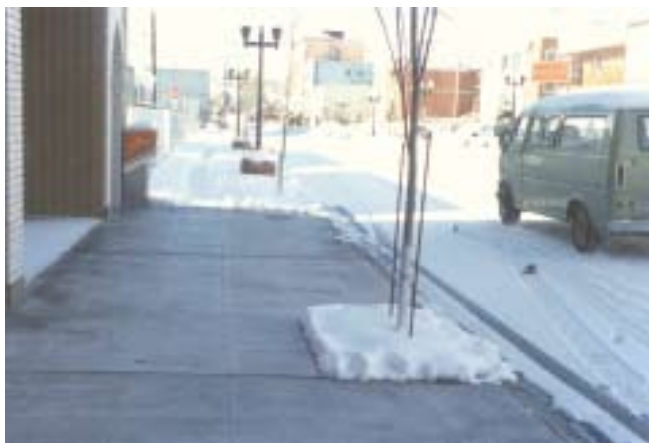
Photo 4: Geothermally Heated Sidewalk Snowmelt (Geo-Heat Center)
