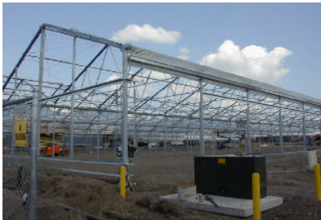
Figure 2. The second greenhouse under construction.
