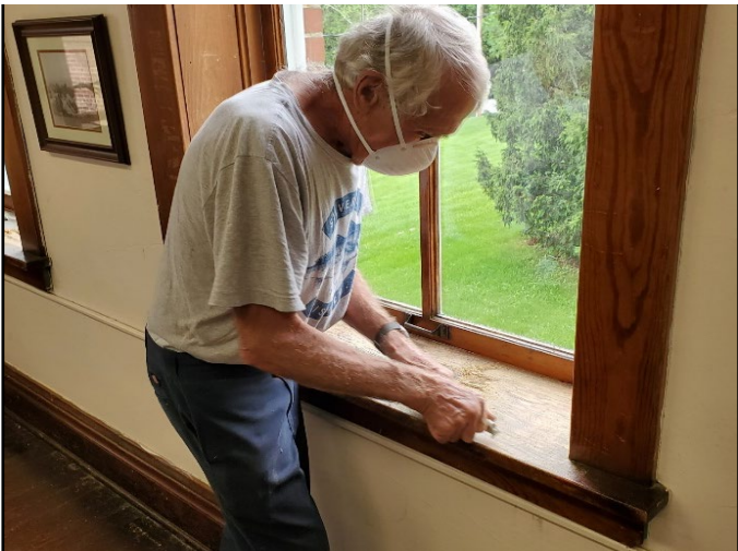
Dan Smith refinishing window frame
