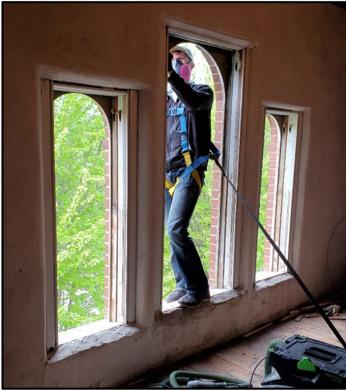
Wadsworth Construction working on attic windows
