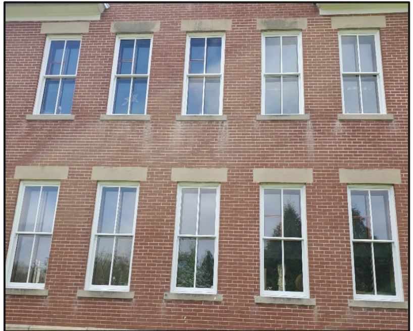
Newly restored frames of double hung windows
