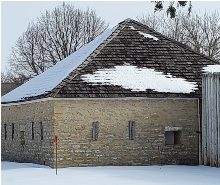
Limestone blockhouse, Fort Atkinson
