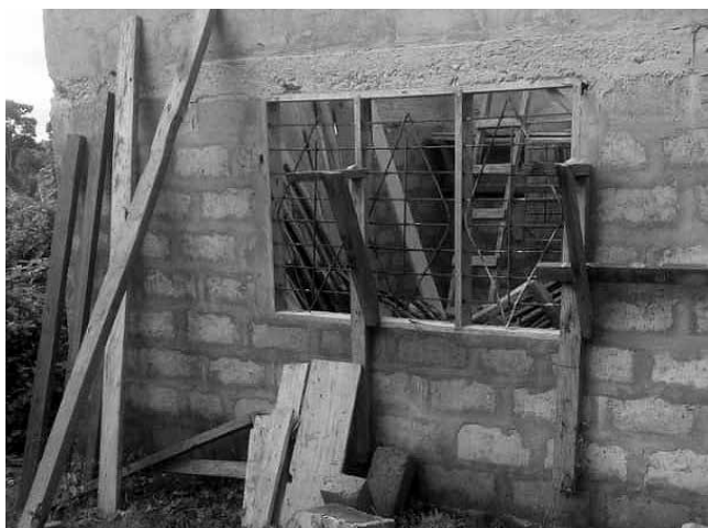
Building work in progress at Akim Batabi School
