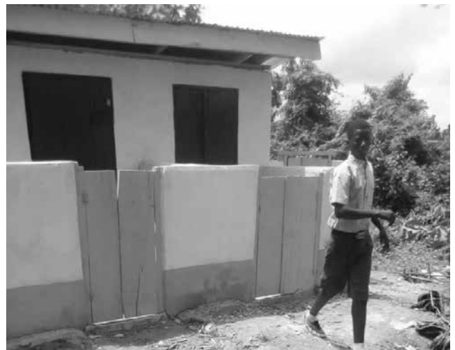
New toilet block at Asanteman Primary JHS
