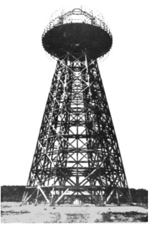
Fig. 3 - Wardenclyffe Tower, part of Tesla's system designed to transmit power across the Atlantic.
