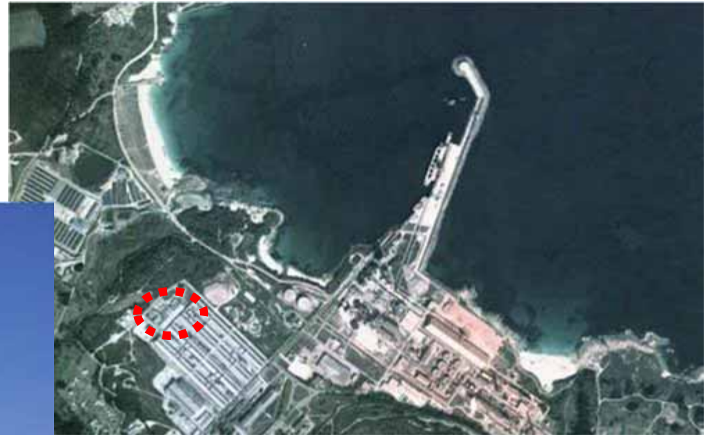
Spain – Biscaya – 420 kV on sea side
