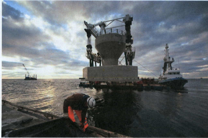
Figure 4 : GBS Lift-off a Construction Barge using Eide 5 Heavy Lift Barge
