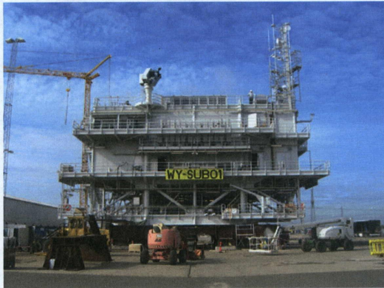
Figure 5 : Substation Assembled in Port
