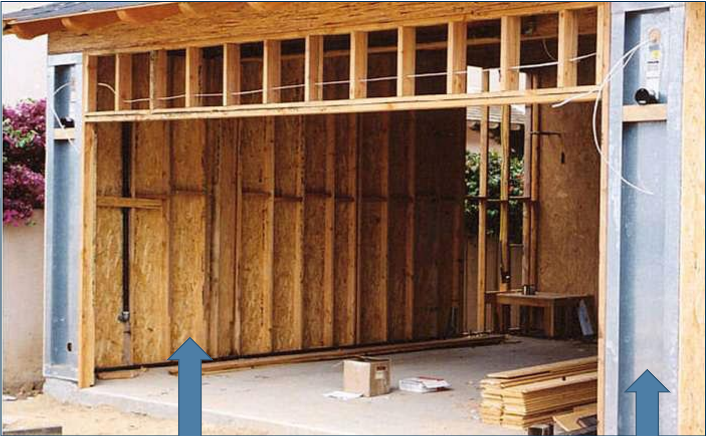
Plywood or OSB on first-floor walls
