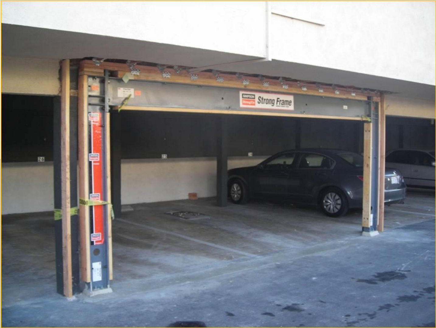
Steel frame around garage door opening
