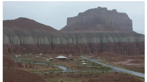
Right: A view of the park's campground, with the combined shower and restroom facility at center.
