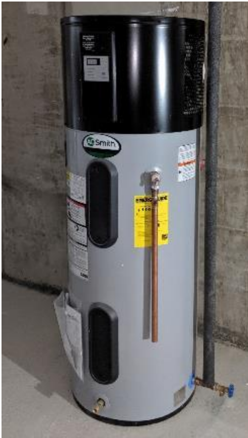
Heat Pump Hot Water Heater
